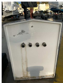
Borne mixte (raccords AEP)
